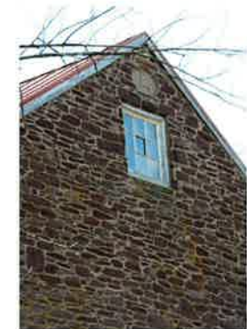
Barn gable with datestone void
