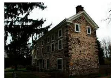
Gable end of main block
