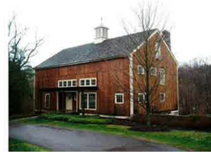
Converted bank barn
