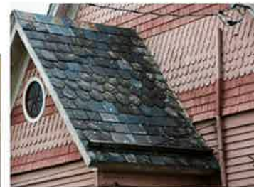
Detail of decorative cladding
