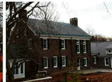
Rear view of house main block
