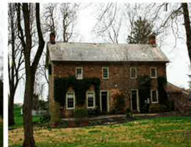
House rear elevation
