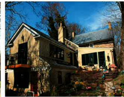
Rear view with modern additions
