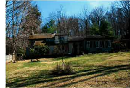
Rear of house
