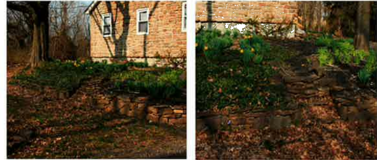
Entry stair & garden wall remains
