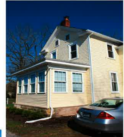
Side view of main block and addition
