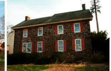
House: rear elevation
