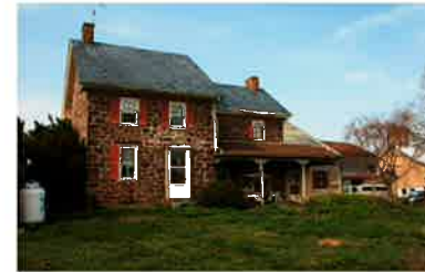
House: front view
