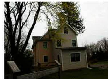
Side view with stucco section at rear
