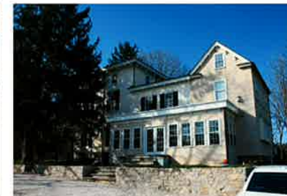
Driveway view (with additions)
