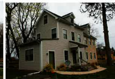
View of wood frame portion
