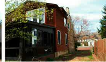
Rear view with rear addition
