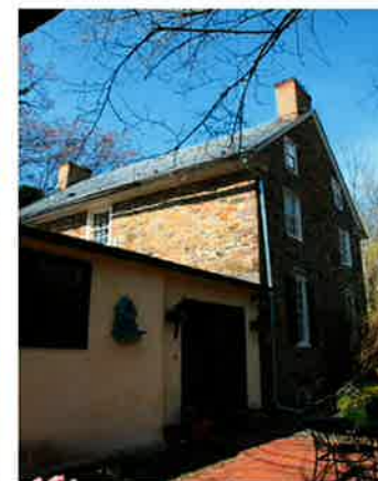
Rear view of main block
