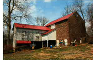
Barn with additions
