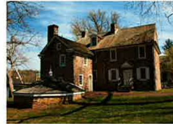
Rear view with ice house in foreground
