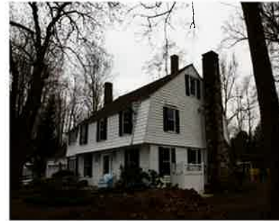
Main block (front view)
