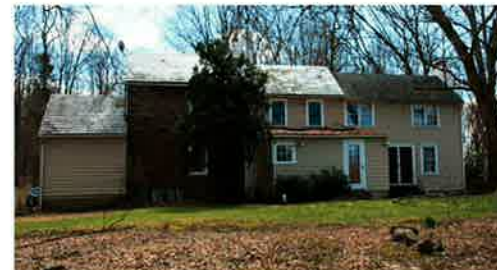
House (rear elevation)
