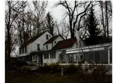
Main block (l) & later additions (rear view)
