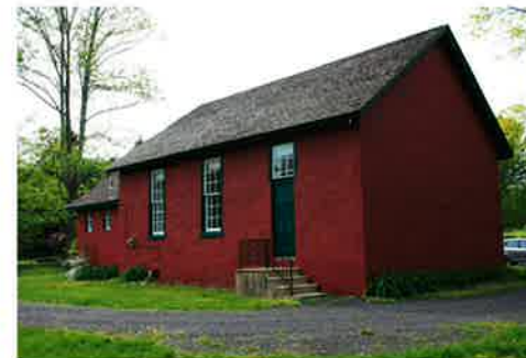
Rear view (with added side entry)
