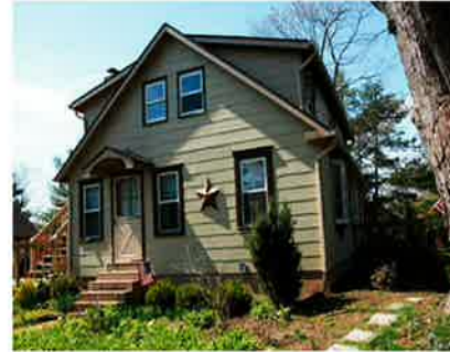
Gable end (view from driveway)
