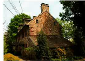
Gable end and house frontage
