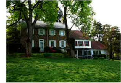
Rear elevation (main block and additions)
