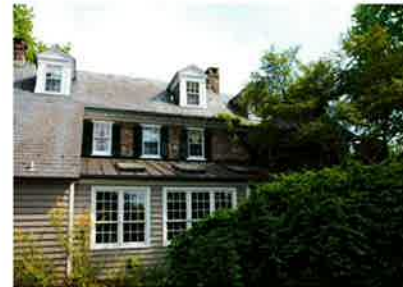
Rear of main block & frame addition
