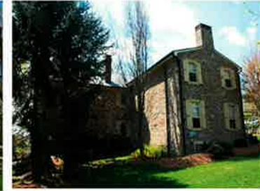
Main block & addition
