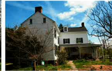
Side view with addition
