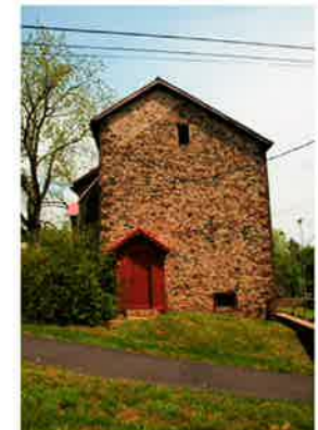
Western end (with change in roofline evident)
