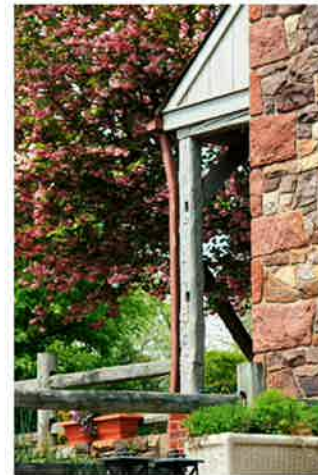
Hewn porch column
