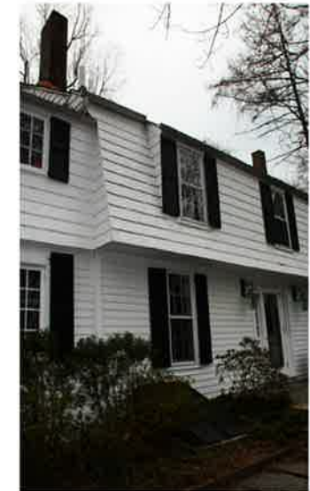
Detail of gambrel roof & dormer
