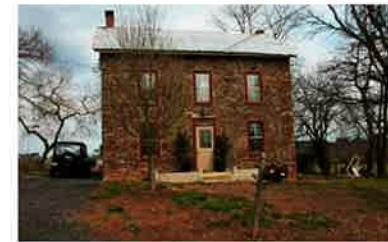
House (street elevation)
