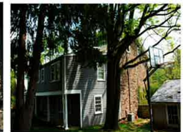
Gable end with frame addition to rear
