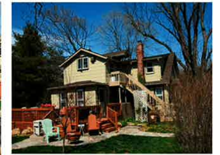
Rear view (with addition)
