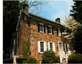
Main block street view
