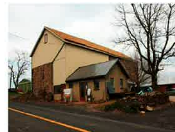
Milk house (foreground) & bank barn
