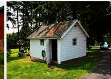
Wood frame shed
