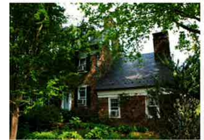
Rear of main block & stone addition
