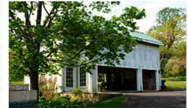
Carriage house (view from driveway)
