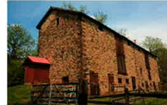
Street view (from west)
