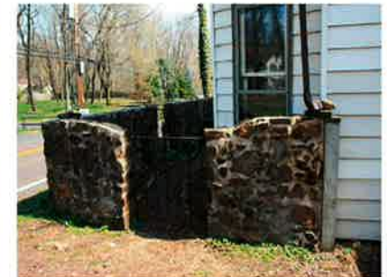
Detail of front wall
