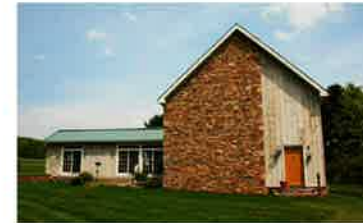
Barn (west elevation)
