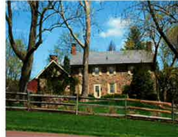
Front elevation with out kitchen in foreground
