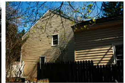
Side view (with main block (I) and addition @)
