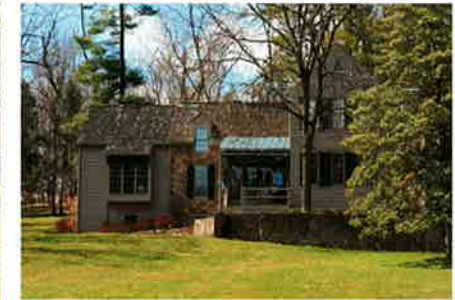
House rear elevation
