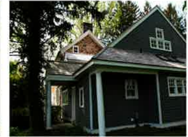
Frame addition to side with main block in background
