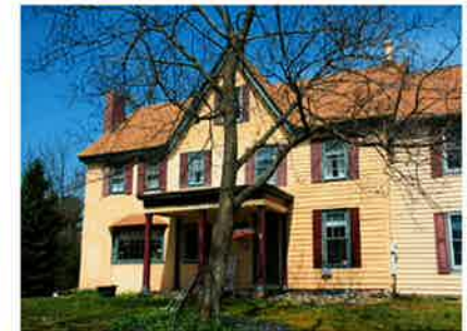
Front view of main block & first
