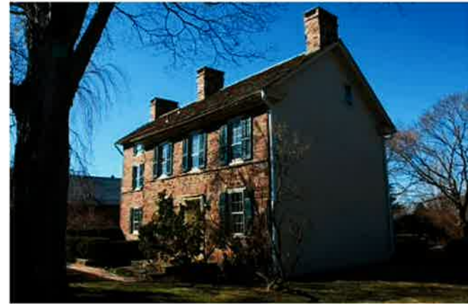
House (street elevation)
