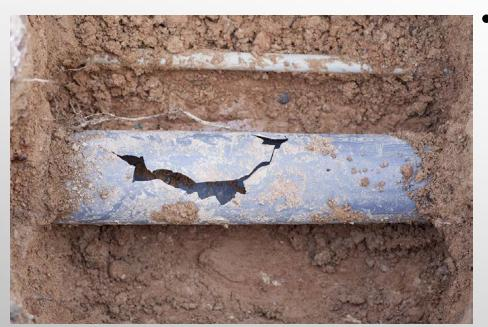
POSSIBLY DUE TO HEAVY SURFACE LOADS (HEAVY VEHICLES) OR TREE ROOT INTRUSIONS OR CLOGS FROM DECAY RESISTANT MATERIALS
