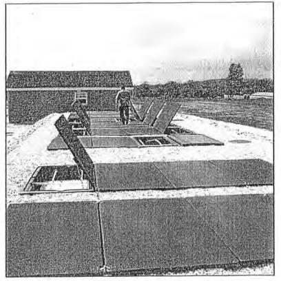
AX100 pods at site 1 (top) and site 2 (bottom) will ultimately serve more than 1,000 new residents of Bethel Heights. Treatment performance remains excellent; after three years of operation, effluent BOD, TSS, and NH<sub>3</sub>-N average <10 mg/L, <10 mg/L, and <5 mg/L, respectively.
