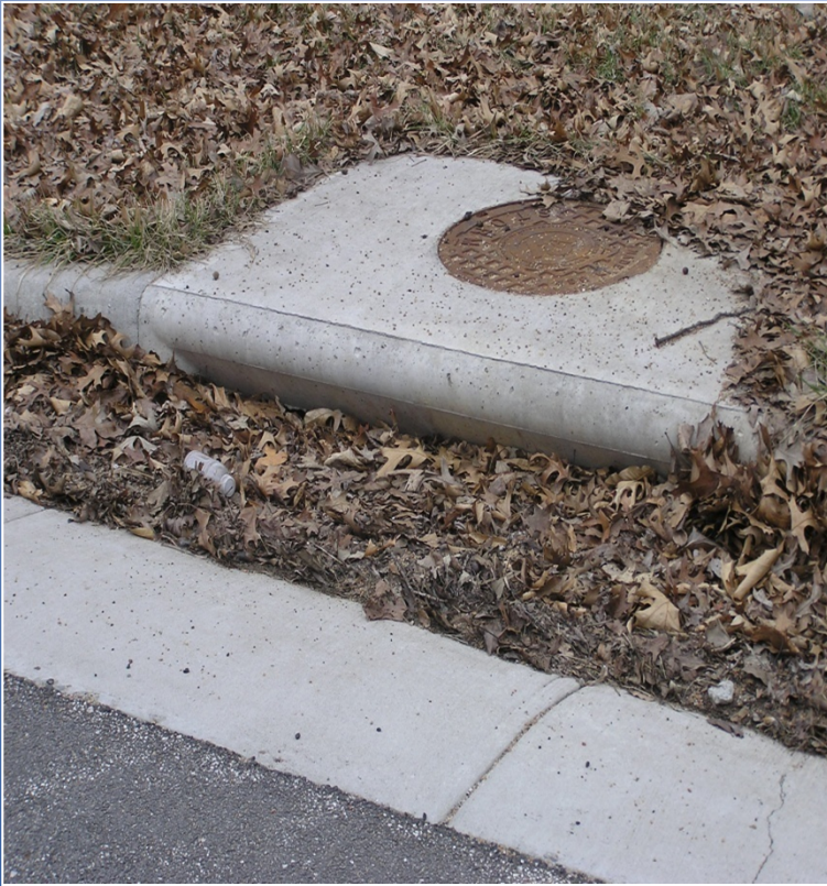
Leaves blocking flow of water into storm drain.
